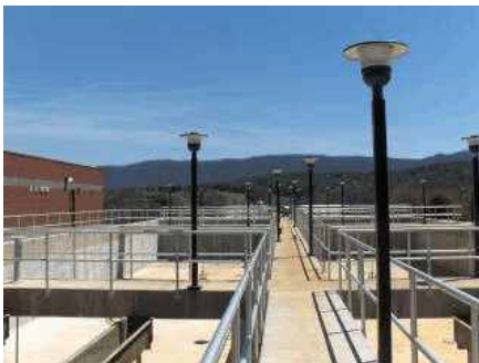
New River Regional Water Plant. Operation will begin in early 2009.
