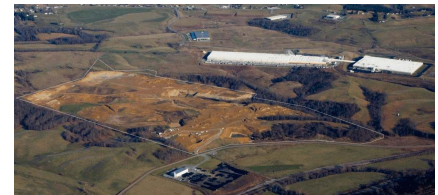
Final year of grading is underway on Lot 24.
