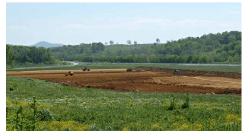
Construction underway on Lot 30
