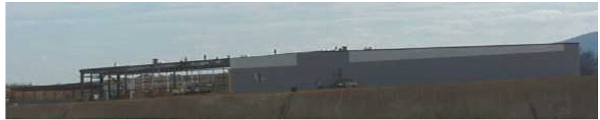
WTI construction progressing.
